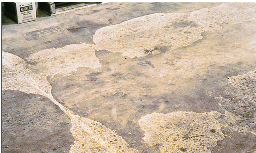
When delaminations form in floors, thin layers of the surface break away from the base concrete. Several factors contribute to the problem.
