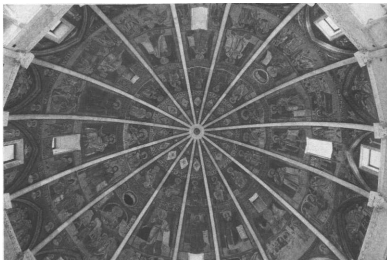
Plate 38 The ribs of the baptistery's vault have no structural function and are supported by the masonry above them. Photo by author
