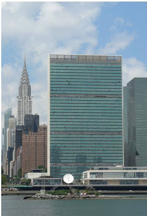
Belmont Island (foreground) is a small artificial island constructed to provide shafts to the 7 Line tunnels under the East River.
