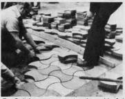
5. Sulphur-concrete paving. Useful not only for building blocks, but also for self-help road building and most other prefabricated concrete applica-
